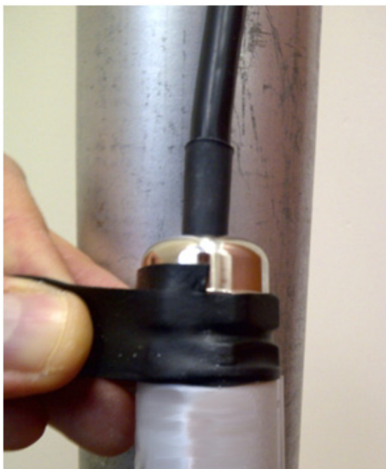
Figure 4-49: Protecting the unit joints with vinyl tape
